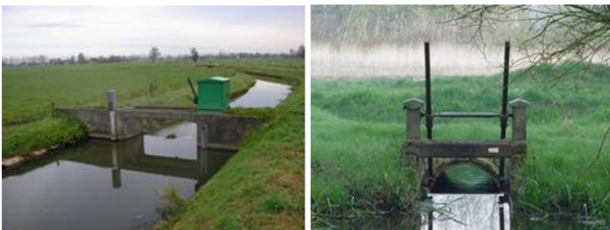
Figure 20 - Small weir (left) and sluice (right)
