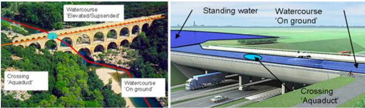
Figure 37 – Aquaduct with two watercourses crossing each other (source: www.leestrainer.nl ) and aquaduct crossing a road (water still on ground level)
